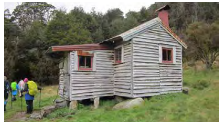
Chaffey Hut, clad in split wood and perched on rock for piles.
